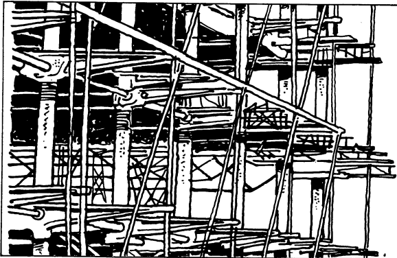
The steel structure is on the outside of the Pompidou Centre.
